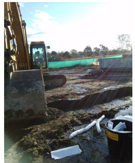
Making a dam with an excavator
